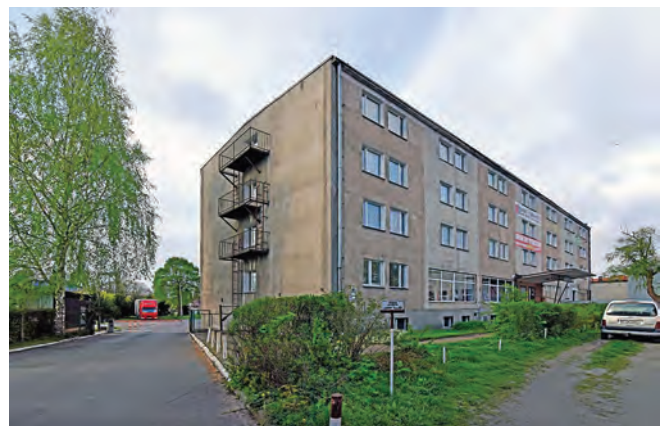
Our 'Communist Era' minimalistic hotel in Świebodzin. Note the lorry with no wheels in the hotel car park and the vertical fire escape ladders. My room was next to the first floor fire escape; the window was blocked by a very large potted plant / bush that was rather too heavy to move in an emergency!
